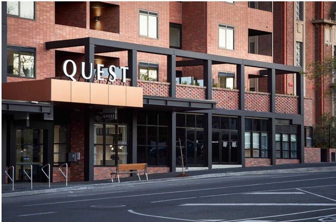
For Peddle Thorp and RPC, being able to merge traditional and contemporary construction techniques was critical to realising their design. While the ground floors are laid in traditional Rustic Red bricks by Lawler Bricklaying, featuring striking hit and miss brick detailing, the upper brick floors are constructed off-site with Brick Inlay, containing matching Rustic Red brick tiles.
