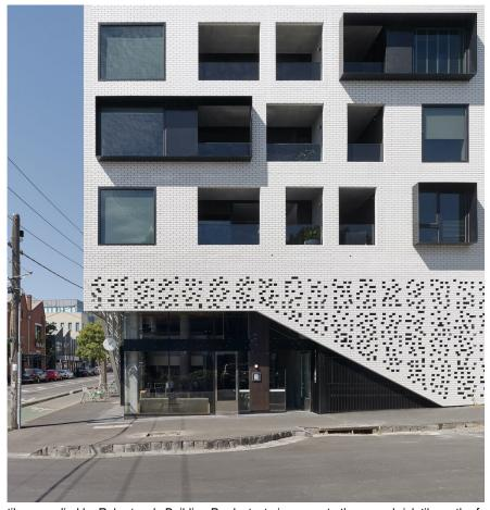
Translating the design into reality was challenging, with its multiple angles for a start, coupled with a custom built breezeway on the ground floor. While the main brick façade was built offsite by the CPP Group, using brick inlay, and delivered ready to install, the breezeway was constructed by tiling brick facings to a steel frame, in situ. This was an absolute labour of love, a work of art, and definitely worth the effort invested. It's simply spectacular.
