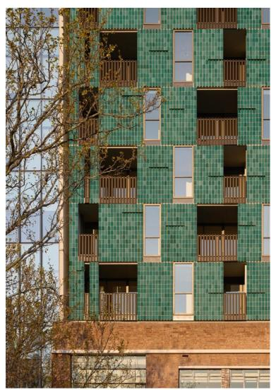
Above the heritage podium sits a tower of concertinaed handmade Rairies Montrieux Jade glazed brick tiles, created with a customised Brick Inlay liner. Using a brick tile was an obvious choice for the tower for its robust qualities and minimal maintenance, given it's a build to rent development, but also to speaks to, and honours, the heritage brick podium.
